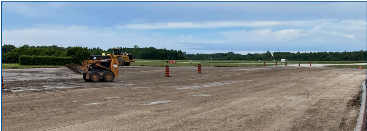
Apron rehabilitation project underway at Goderich Regional Airport, ON
