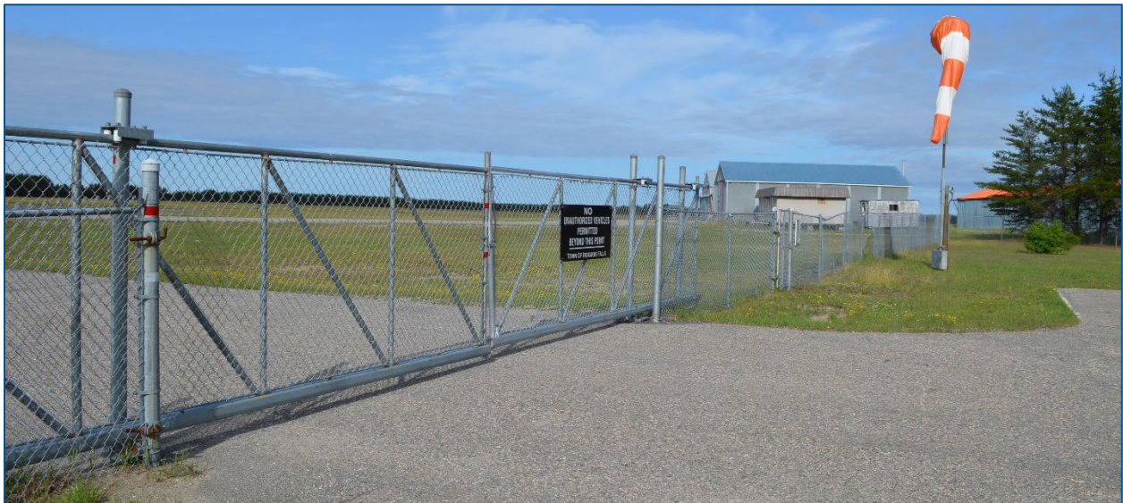
Perimeter access controls and wind direction indicator at Iroquois Falls Airport, ON
