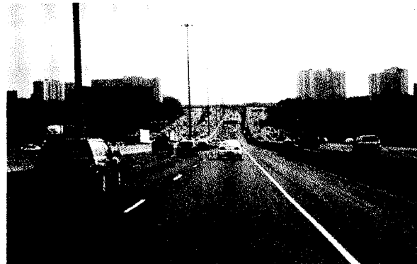
Highway 401 through the City of Toronto
