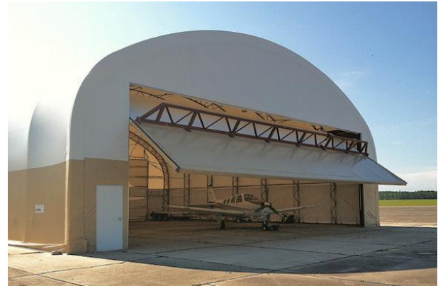
A steel-framed, fabric covered hangar with a hydraulic swing-up door.
