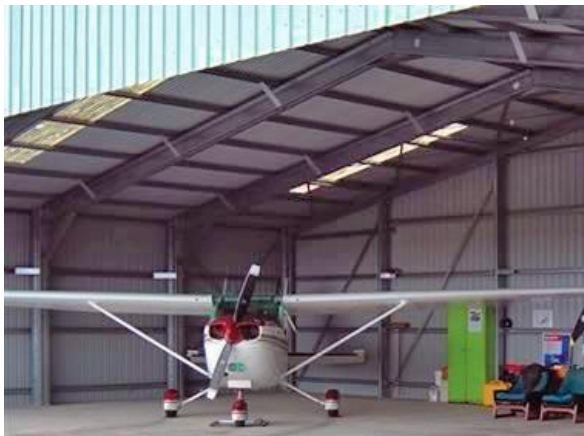
The steel structure of a steel-framed hangar visible from the inside.
