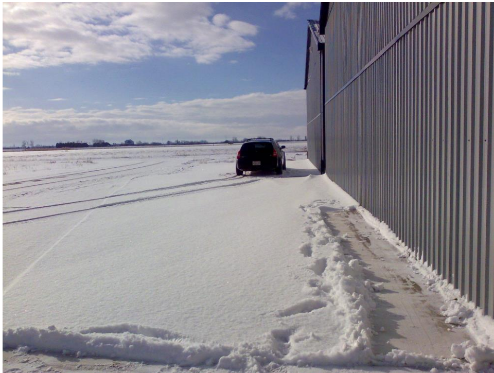
Example of roof sloping away from hangar doors, if not a large overhang is required.
