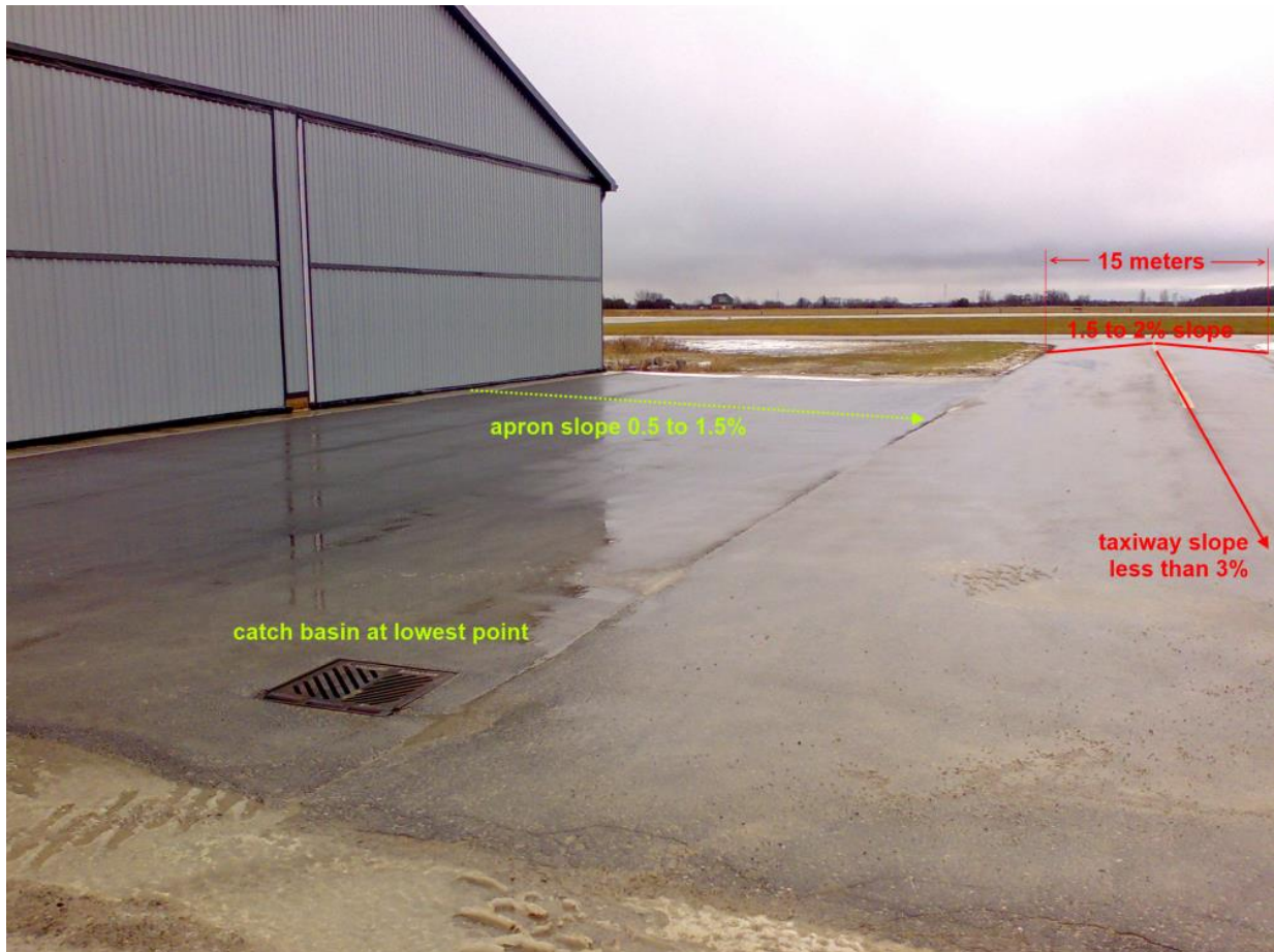
A taxiway and apron draining to an airport storm drainage system.
